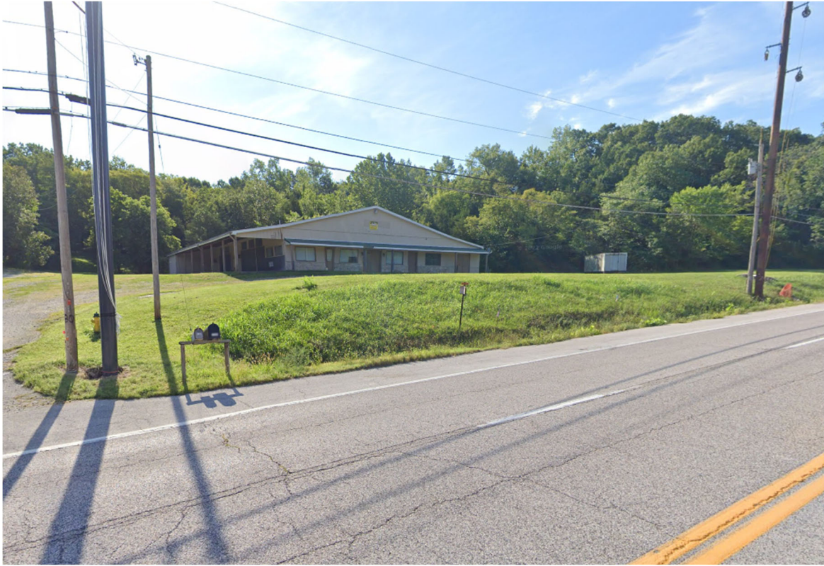
STREETVIEW FROM HWY 61/67 (AUGUST 2022)
